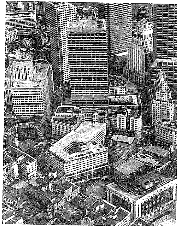
1981 - Twelve decades later every single building but one—the Old South Meeting House at far left—is gone. What the great fire of 1872 did not take, real estate pressures did. But the streets are entirely intact, and buildings like the parking lot bent in the middle foreground and the Shawmut Bank building tall and trapezoidal in the middle top, must twist to fit the streets and their angular lots. Milk Street is the curving street on the left; Franklin curves on the right. Washington Street angles down in the foreground from the Old South Meeting House.
